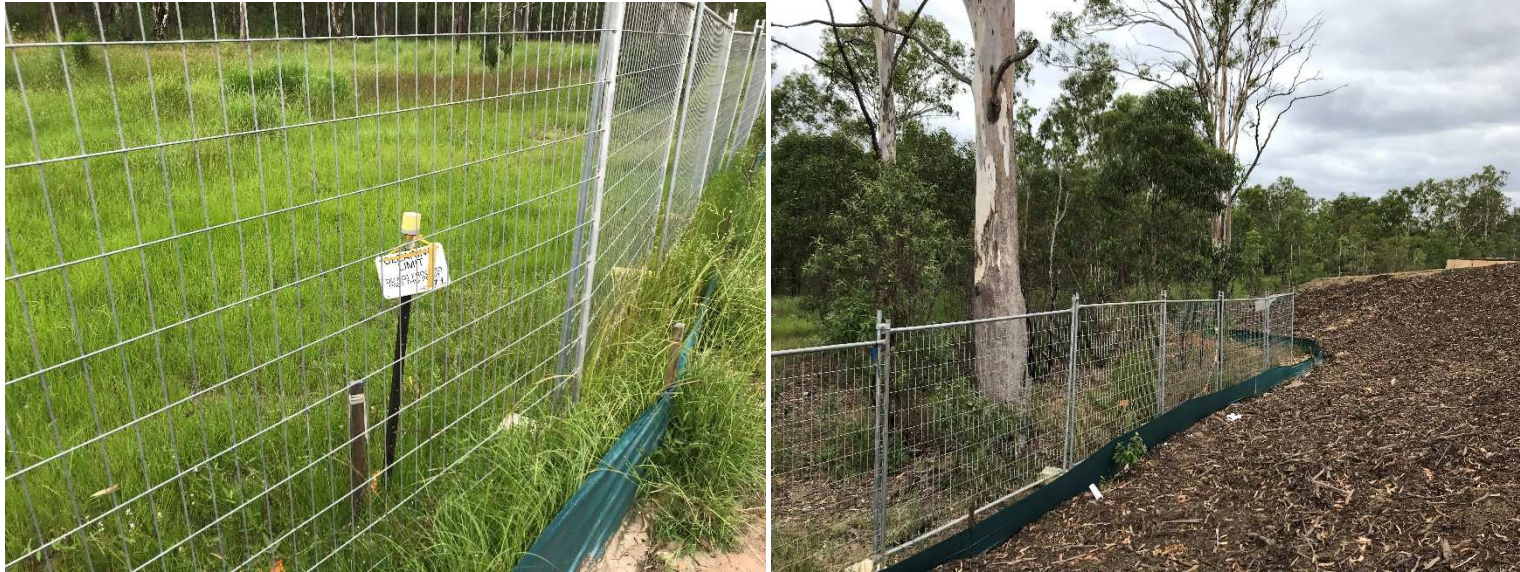
Photo Plate 2: Demarcation of clearing extent with steel fencing and signage.
